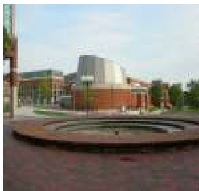
New Magruder Hall extension, completed last year.
